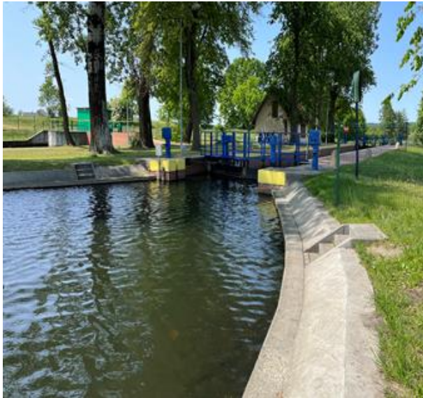
Figure 10. Site 5 Noteć Canal – Łochowo. A view to upstream of the lock (own picture).
