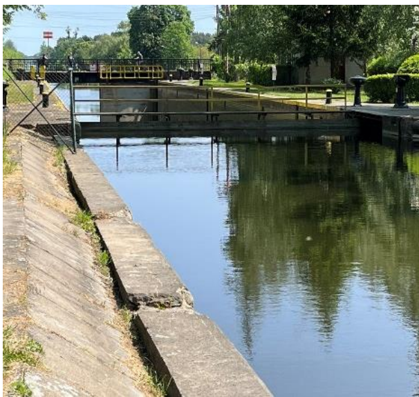
Figure 7. Site 3 Prądy. A view to upstream of the lock (own picture).
